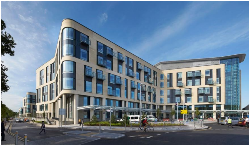
^^ Main Southmead Hospital building
